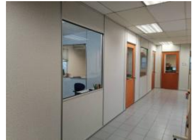
After: Partitioned offices
